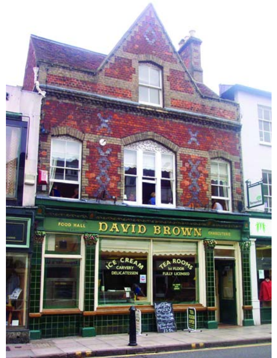
Fig 8: The fascia is the correct depth for the shopfront and the lettering sits well within the frame. The colour scheme is subtle and unifies the whole front - including the door. The stallriser is an appropriate depth.
