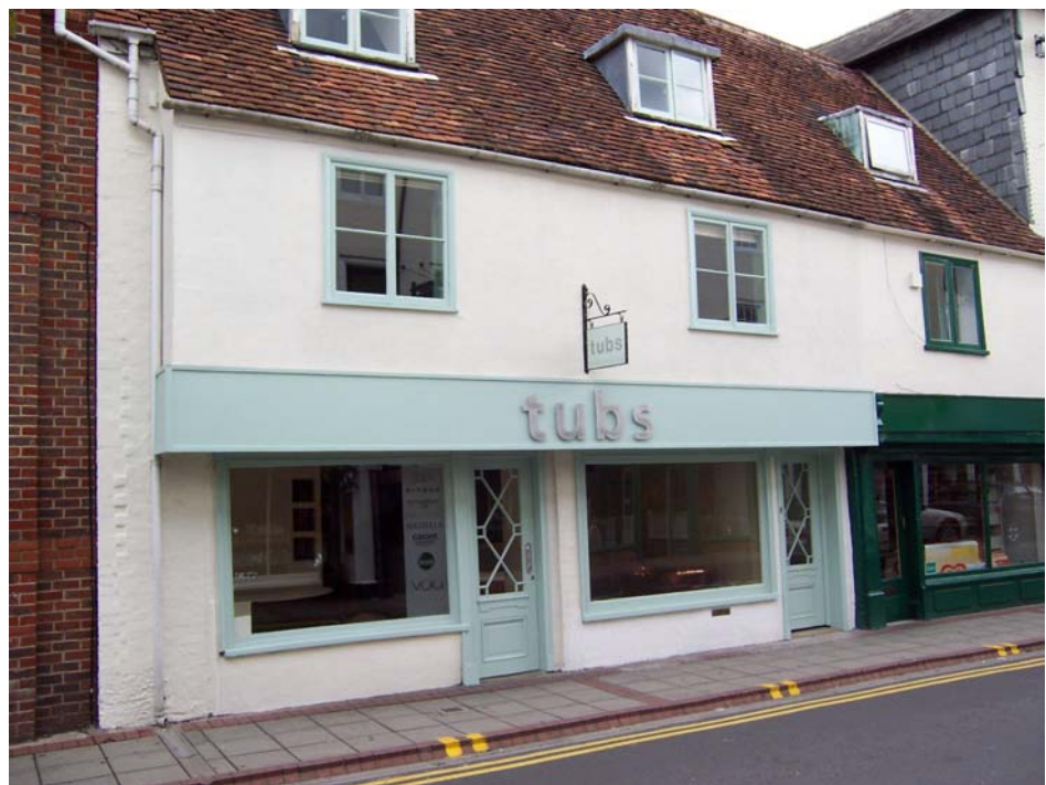
Fig 12: Although in this case the letters are shiny metal, due to the brevity of the word and the simplicity of the style - a subtle, attractive fascia is achieved.
