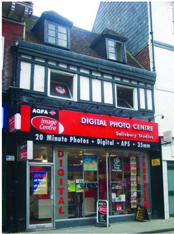
Fig 7: This fascia is too large for the shop and is made of shiny modern materials. The red is garish and too much text is crammed onto the fascia so that it has a confused and 'busy' appearance. The modern aluminium' shop front is not in keeping with the building above. A deeper stallriser would also have been preferable.
