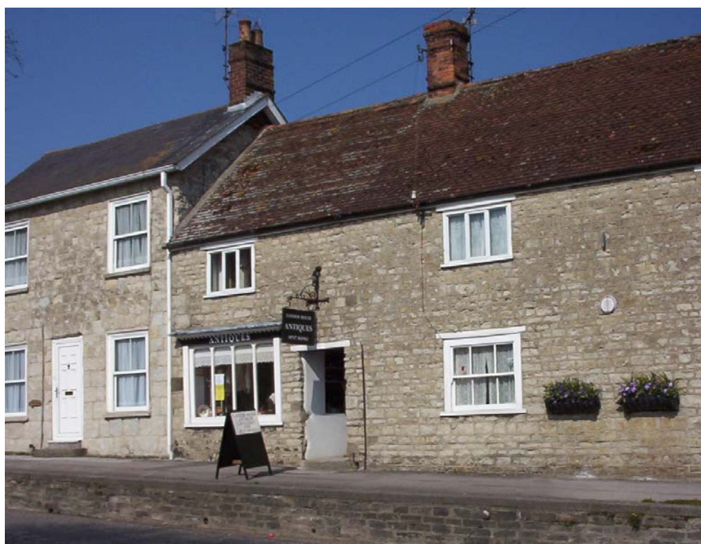
Fig 5: An attractive shop in mainly residential area. The 'low key' commercial approach suits the setting.
