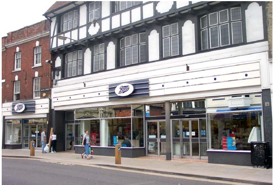
Fig 11: A shopfront with a wide expanse of flat glass. The fascia is made of modern materials and is overly large, impinging on the first floor. The shopfront does not reflect the architecture and the rhythm of the upper floors and the fascia is overbearing.
